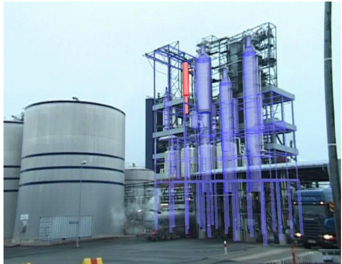
Figure 1. Example of Augmented Reality on an industrial plant
